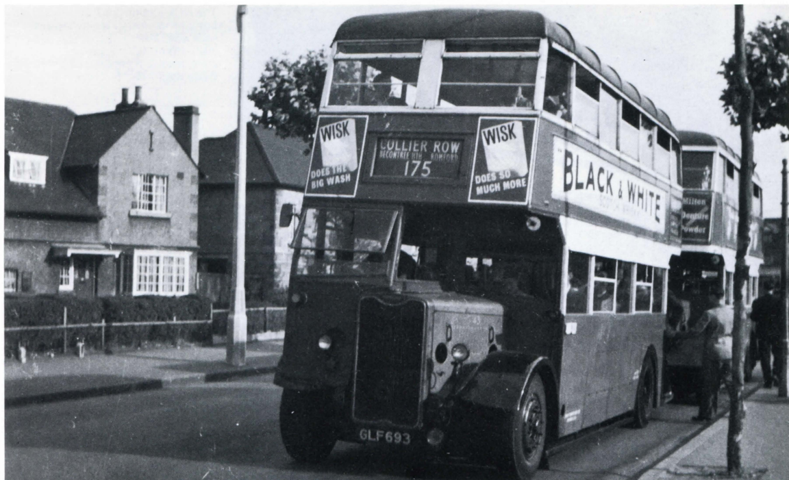
G43 was unique in being the only London Guy to have a Duple body. The wide central panel between the front upper deck windows is clearly visible. Route 175 worked in extremis between Stapleford Abbotts and Poplar although through journeys were rare. In this July 1949 view a short is being worked by Upton Park to Collier Row. Alan B. Cross
