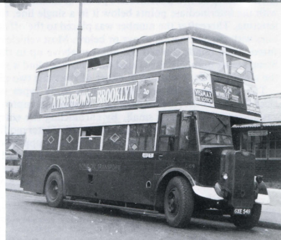
Right: The diamond openings in the window maskings are clearly seen as G109 awaits a duty on route 92A during the war. The protruding radiator indicates an Arab II. Hanwell operated Bs as well as Gs and was the only garage to operate two utility classes. J.F. Higham
