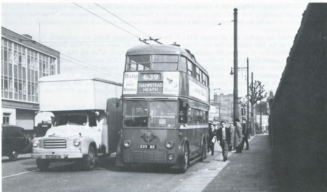
Top left: A load of passengers have disembarked from L3 1424 at the Parliament Hill Fields terminus of route 615 and the driver prepares to make the U-turn across the Swains Lane junction, for the protection of which manoeuvre a 'DANGER' sign was displayed in the frame of an old 'shamrock' type tram stop frame in West Hill. Ken Glazier. Top right: The World Of Suzie Wong is on at the Plaza, Regent Street but it will not be the world of the 653 much longer. L3 class 1394 shares the dilapidated background of Aldgate lay-by with an RT during January. Ken Glazier. Above: All-Leyland K1 1062 prepares to make the descent of Pentonville Road to Kings Cross on route 639. Michael Dryhurst.
