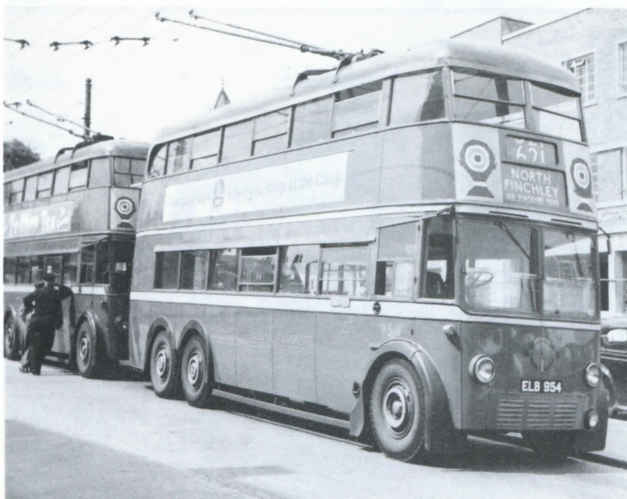
The other L2 withdrawn in April was the prototype (954), new in 1938. It had a shallower windscreen than the production vehicles and this gave it its most distinctive feature, the continuation of its lower cream band around the front. Ken Glazier.
