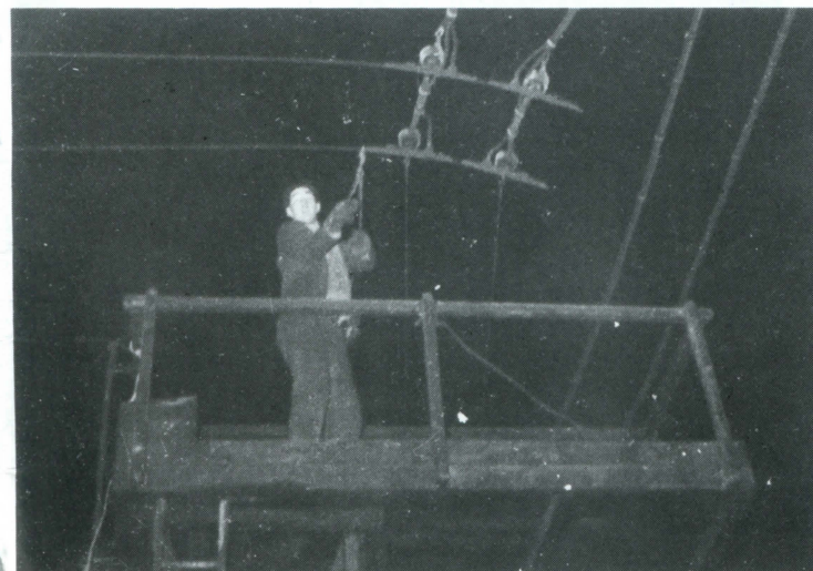
The wires are partly cut at Colindale as another of Mr Cohen's employees prepares to make the next cut, on 10th March 1962. Hugh Taylor
