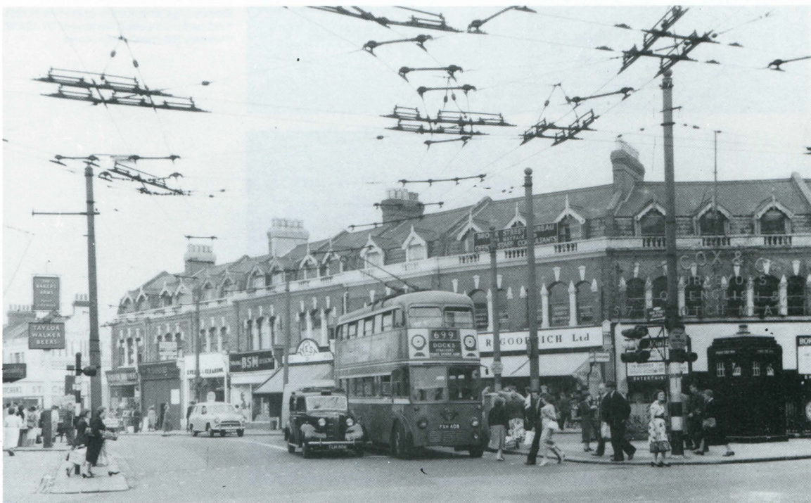
Below: Major junctions hosted great weights of overhead: that at 'Bakers Arms' Leyton weighed about three tons for the whole layout (excluding Lea Bridge Depot). Here 1406 waits beneath a large proportion of that weight. As the conversion programme spread, redundant junctions were removed at such locations as this, making life easier for remaining routes. C Carter
