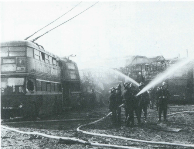
A few fires occurred at Colindale, the worst occurring in August 1960 when a number of vehicles were completely burnt out. The firemen seem to be enjoying themselves in this photo. Hendon and Mill Times
