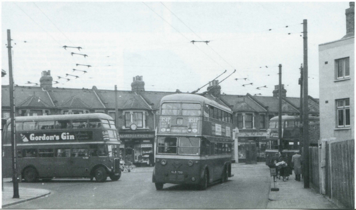
STAGE 3: Hainault Street at Ilford was wired as late as 1958 due to the rebuilding of Ilford Station Bridge. 1759, an SA3 originally bound for Johannesburg, enters this thoroughfare. The bamboo pole hanging from the traction standard, which has no finial, is for easy access and indicates that dewirements often occurred there. C. Carter
