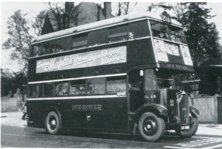
Red Rover's fine Birch bodied Lance was new in August 1932, and contrary to general practice was transferred to PB virtually unaltered as DL28 from March 1934. The minute side-lamps were unchanged – there were no headlamps – and the all-over dark red livery stayed smart until repainting in standard colours late in 1934. D. W. K. Jones
