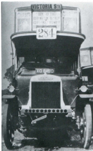
Right: The full frontal view of XO 8490 (26) obtained in July 1927 shows the 11-hole frame cross-member and wider frames that distinguished the LB2 from its successor marks LB4 and LB5. W. Noel Jackson Far right: The LB4 is exemplified here in 1930 by XP 7074 (21, ex-Public 21) which provides a contrast with the previous photograph. The narrower frame width gave a better steering lock. W. Noel Jackson
